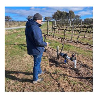
Twelve Tempus® Ag 1-station LoRa radio battery controllers were placed at twelve 50mm field valves with DC coils. One Tempus® Ag battery controller is connected to a flow meter and another is connected to a fertigation pump. A Tempus® Ag latching pump relay is connected to the vineyard's variable speed pump.
